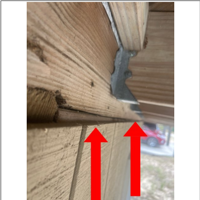
No flashing installed above the upper edge ground floor SSE exterior siding. To ensure moisture cannot penetrate at this location, a licensed general contractor should evalaute and make any necessary corrective actions
