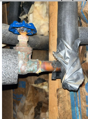
Main water shutoff is located within water meter enclosure at the SW corner of the property
