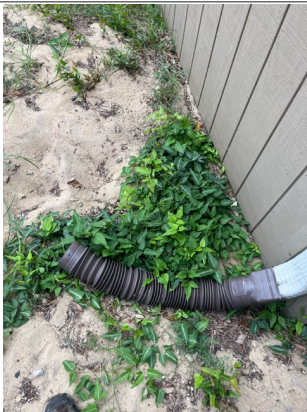
Due to the negative grade, NE corner Downspout terminates at the base of the home. While an extender is currently installed, it likely terminates runoff that pools against the home. A licensed gutter technician should evaluate termination point to be extended.
