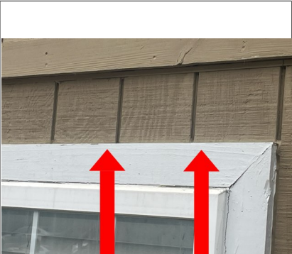
"Z" Flashing not installed at the upper edges of trim above horizontal trim, windows and doors at the exterior. To ensure moisture cannot penetrate and these upper edges, a licensed repair professional should evaluate condition at these edges and consider adding this flashing where neccesary as an upgrade
