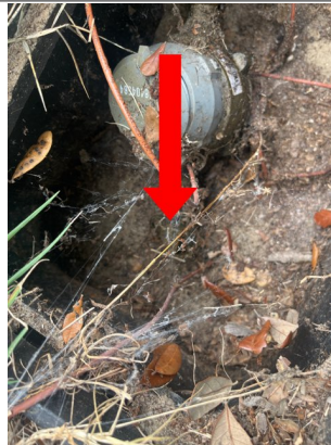
Main water shutoff is located within water meter enclosure at the SW corner of the property
