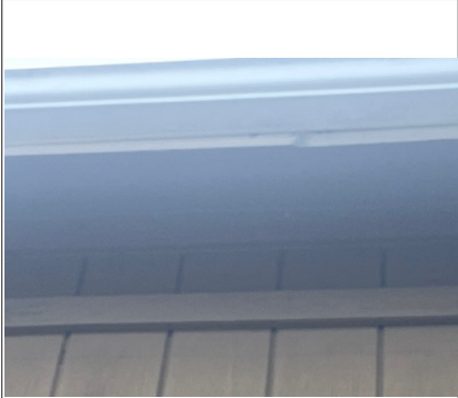
No flashing installed above the upper edge ground floor SSE exterior siding. To ensure moisture cannot penetrate at this location, a licensed general contractor should evalaute and make any necessary corrective actions
